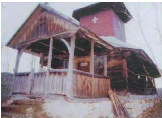
Fig. 4. The wooden church from Bozioru de Sus.
