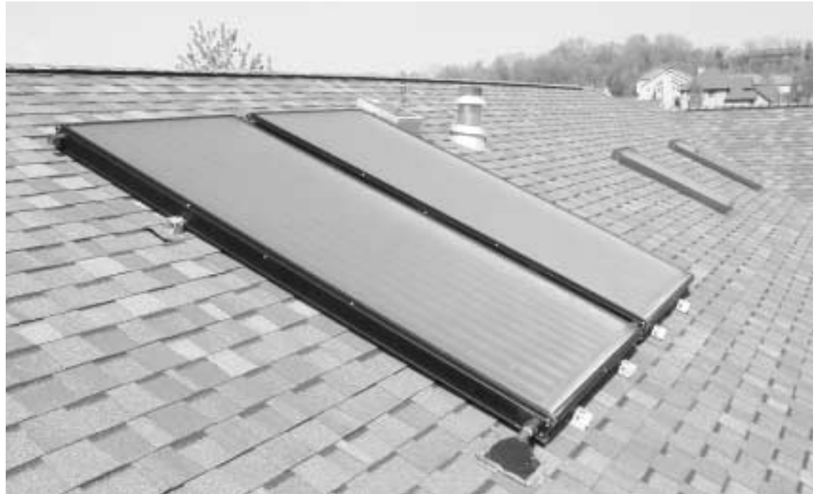
Solar water heating panels attractively integrated into the roof of a house.
