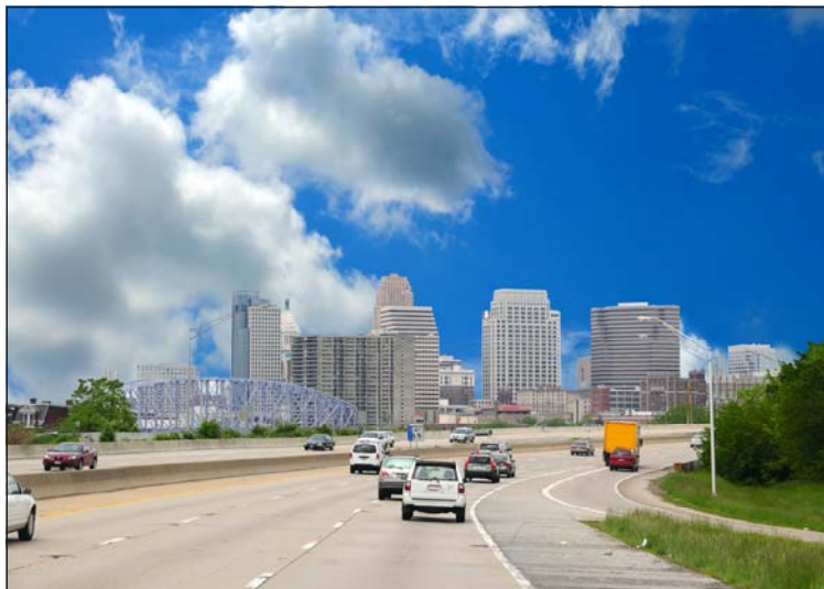
Figure 1. Our economy depends on transportation infrastructure. We drive to work and school on roads each day. Most of our food, clothing and consumer products are delivered in trucks that travel our interstate highway system.
